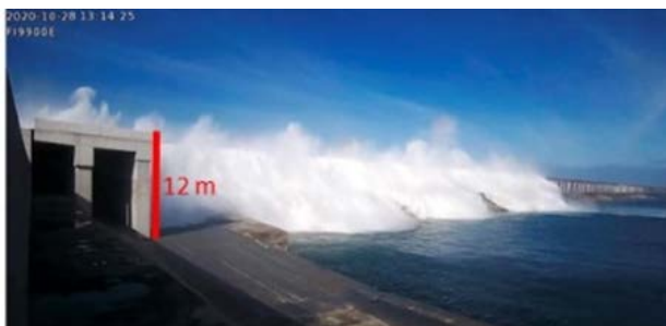
Figure 8 - Overtopping event (date: 28/10/2020)
