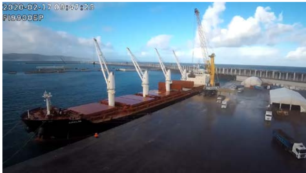
Figure 3 - Moored ship close to the 3.3km main breakwater.
