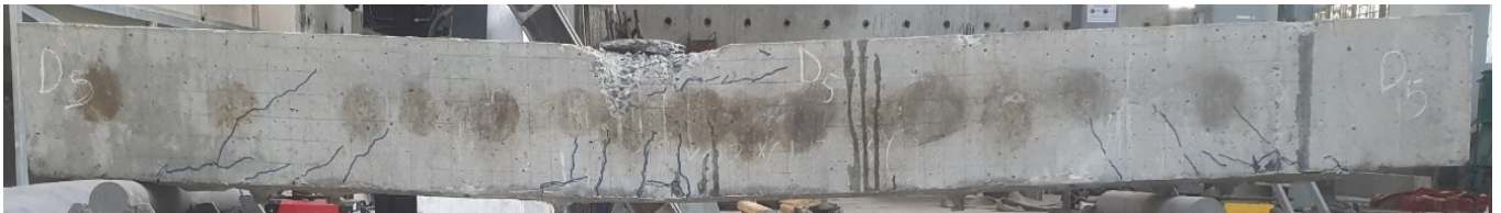
(f) Rupture type of D5: Slip failure at the left end.
