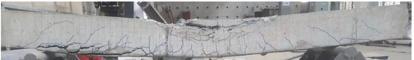
(g) Rupture type of D6: Slip failure at the left end.
