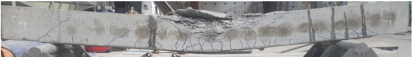
(e) Rupture type of D4: Slip failure at middle.
