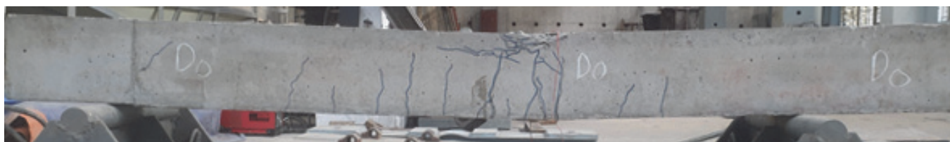
(a) Failure mode of beam D0: Ductile failure at midspan.
