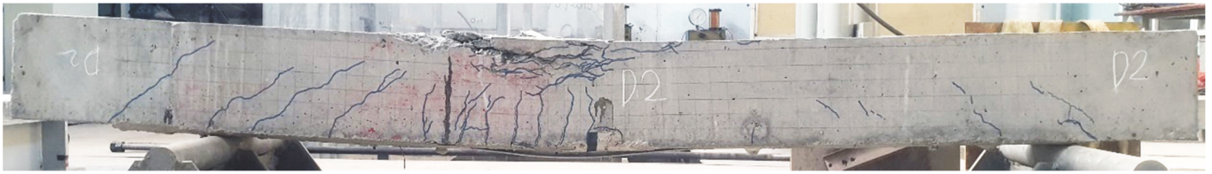
(c) Rupture type of D2: Slip failure at middle.
