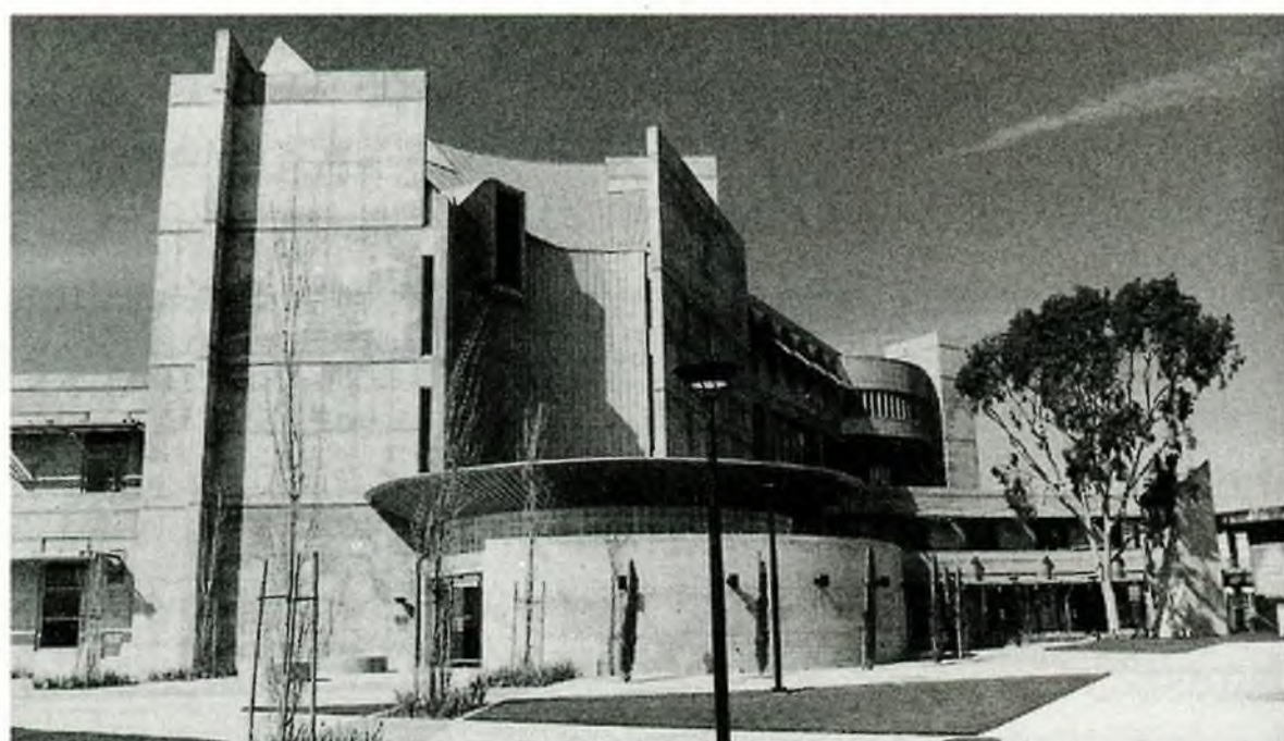
To blend in with surrounding architecture, the new Learning Resource Center at San Diego Mesa College, designed by M.W. Steele Group, Inc., is a poured-in-place concrete structure, affording a naturally quiet environment.
