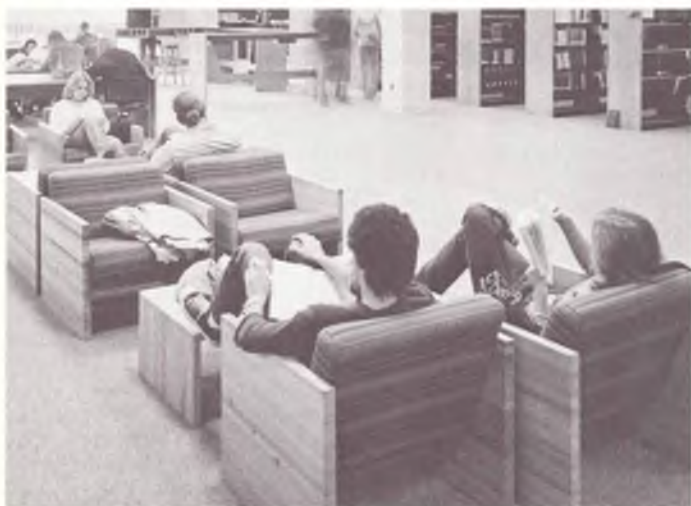
Exterior and interior views of new Ramapo College Library.
