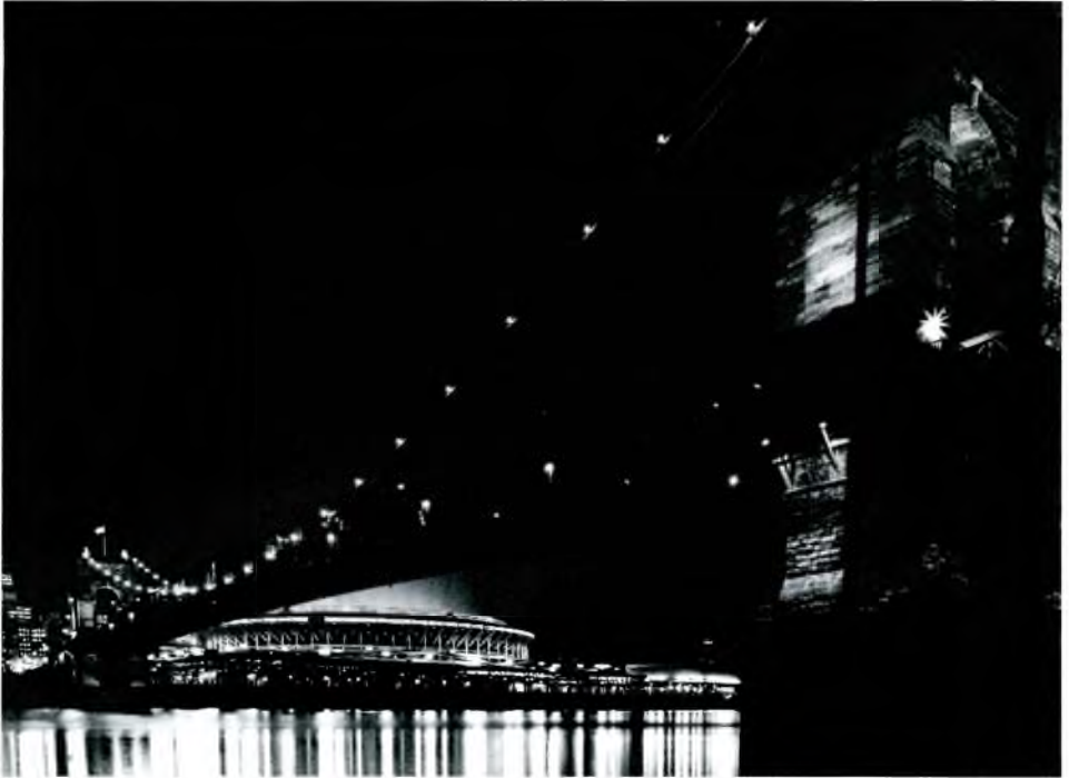
The graceful span of the John A. Roebling Suspension Bridge is a contrast of Old World charm against the skyline of downtown Cincinnati.
