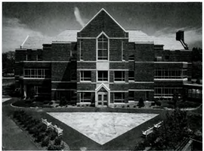
The new 84,500-square-foot Boston College Law School Library is fully wired with power and data hook-ups for every reading table, study carrel, window bench, and group study and lounge seat within the facility.
