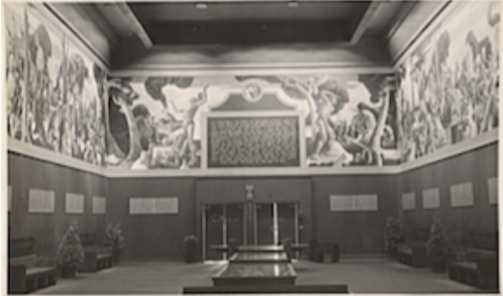
Figure 9. Indiana Hall interior facing west, towards entrance, (1933), photograph, Wallace Richards Papers, Archives of American Art, Smithsonian Institution
