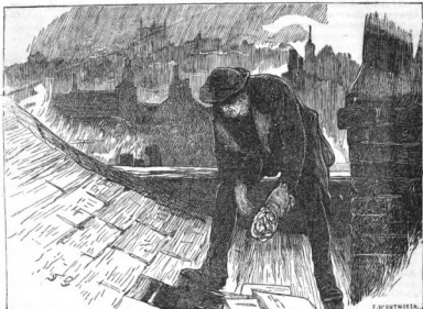
"HE PLACED THE PRECIOUS PARCEL WITHIN THE ROOF."
