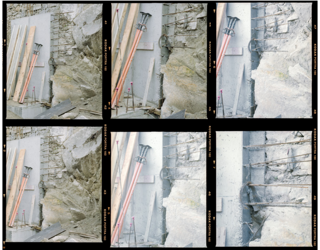
2. Contact sheet. April 20, 2019. São Vicente, Braga. Sequence at a construction site.
