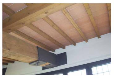
Figure 6. The ventilated roof structure.
