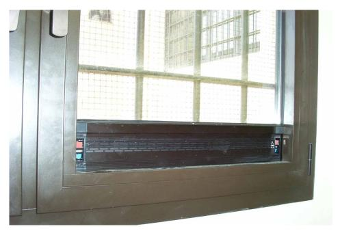
Figure 17. The special grids integrated in the windows frame.
