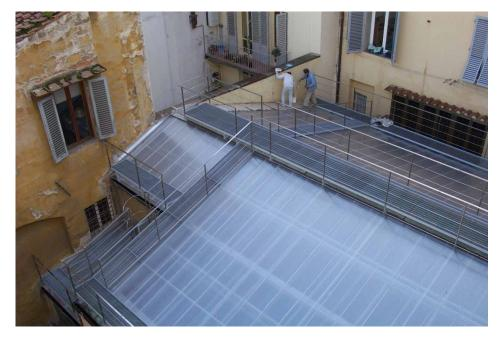
Figure 14. The new skylight: external view.
