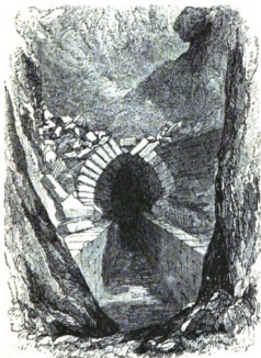
Vaulted Drain beneath South-east Palace. (Nimroud.)
