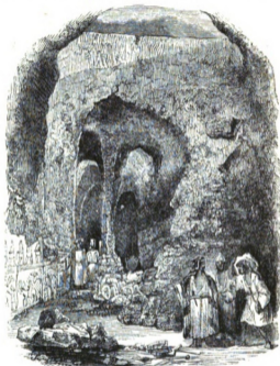
Underground Excavations at Kouyunjik.
