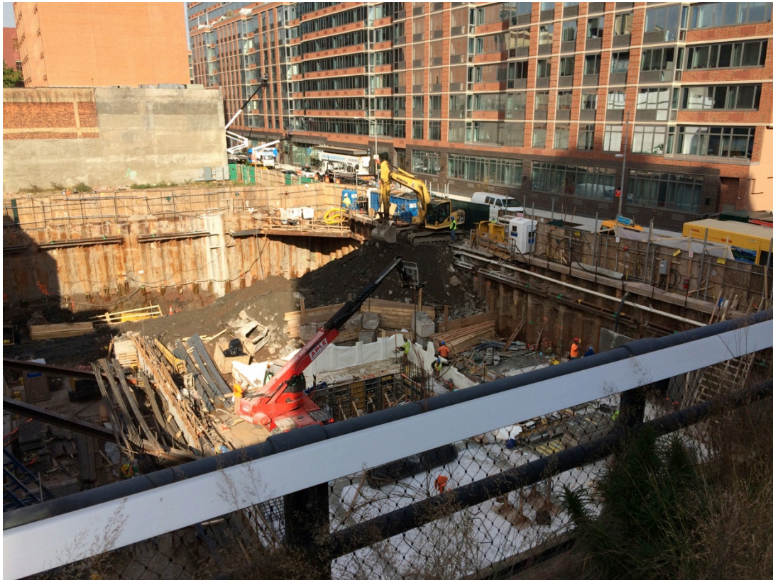
Figure 21 Building site in Chelsea, Manhattan 2014
