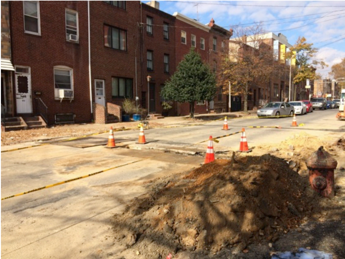
Figure 96 Road works outside Crane Old School Studios, Philadelphia 2014
