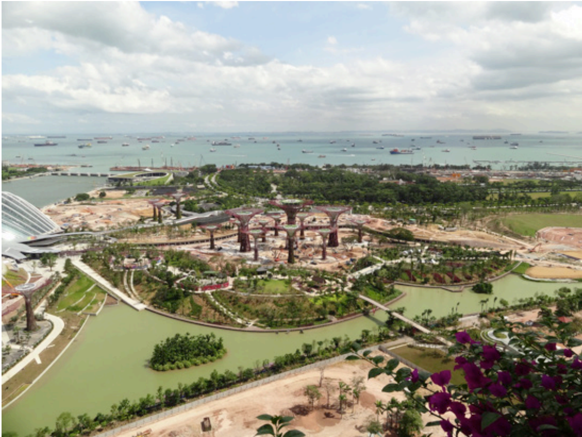
Figure 59 Gardens by the Bay construction site Singapore 2012
