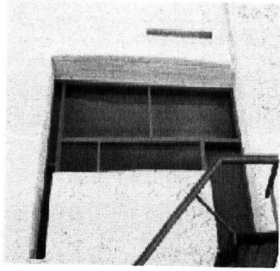
Figure 7: Second-storey exit, north wall
