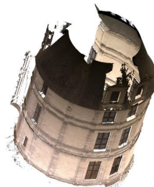
Figure 11: 3D point cloud of Tour du Donjon (TO)
