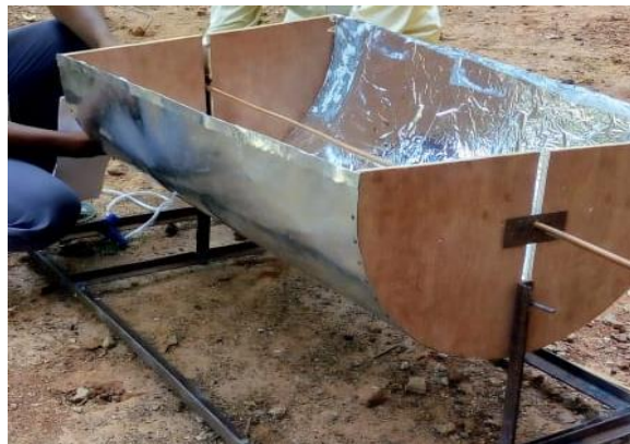
Fig.2:-Fabrication of solar parabolic trough collector
