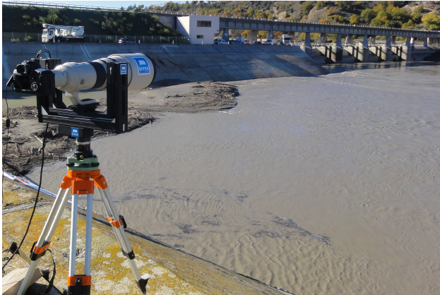
Figure 6. High resolution camera, 600 mm lens and panoramic head facing upstream wall of a dam
