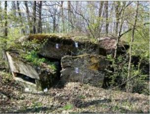
Figure 8. Image of pillbox № 451 with coded targets
