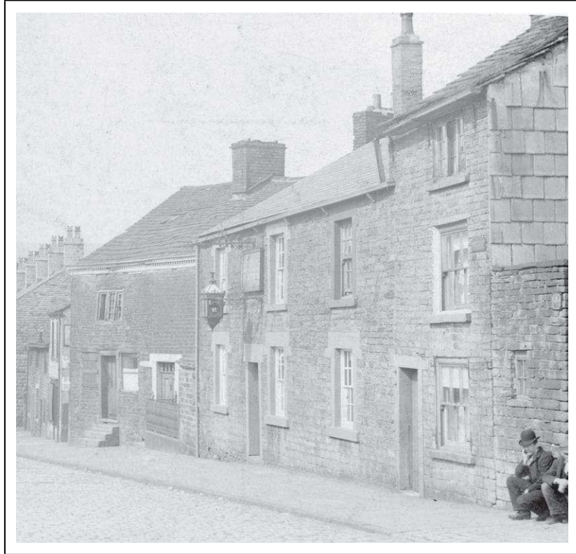
Figure 5. Incremental Development. Building A with three steps predates the rebuilding, appearing on a lease plan of 1789 as a saddler's shop and is part of Chain 276. The property which extends it, B, is accounted for within Chain 38, its construction presumably corresponding to an increase in its annual value of £1 in 1792, or a further increase of £1 in 1793. Property C occupies a site accounted for within Chain 40. A notional value of £1.50 in 1784 increased to £3 by 1792, and £3.50 by 1806. The site was granted a 99-year lease in 1796, including an area where development had taken already taken place (Source: Tameside Image Archive; Copyright Tameside MBC).
