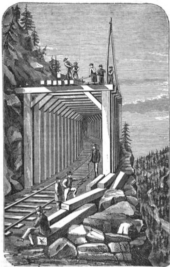
Constructing Snow Sheds, Sierra Nevada Mountains, C. P. R. R. See page 164.
